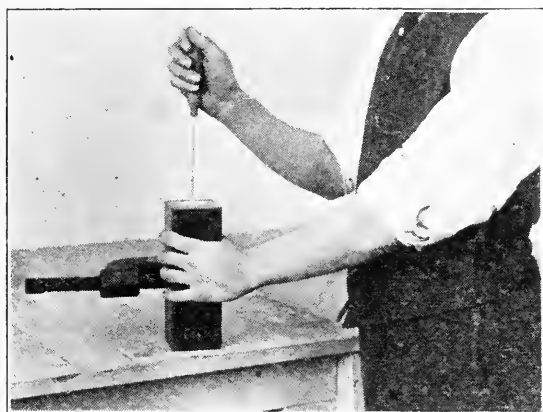
FIG. 536. CORE-BOX IN USE.
